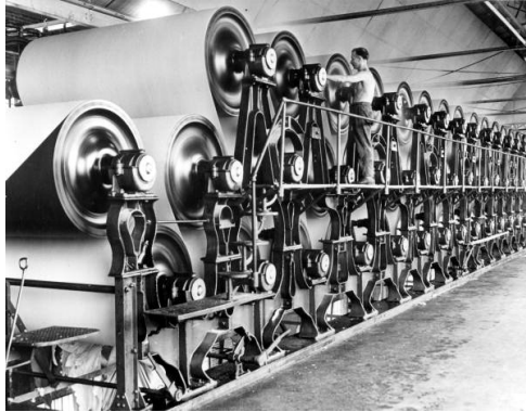
Figure: A paper web being driven through a paper machine.
