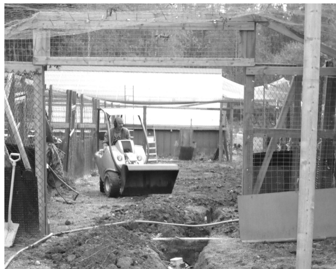
Fig 5. The AVANT 220 installing piping and electricity for Hall 3
