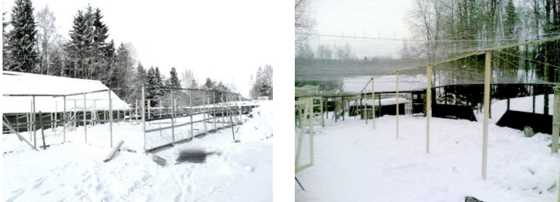
Fig.3. -4. New walls 200 m and new roofs over 2000 m 2 .
